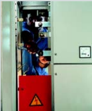
Wide 250mm Cable alley makes cable termination easy.
